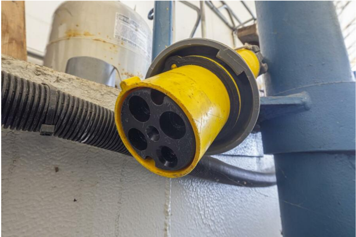
Shore-power 100amp Shore-power connection
