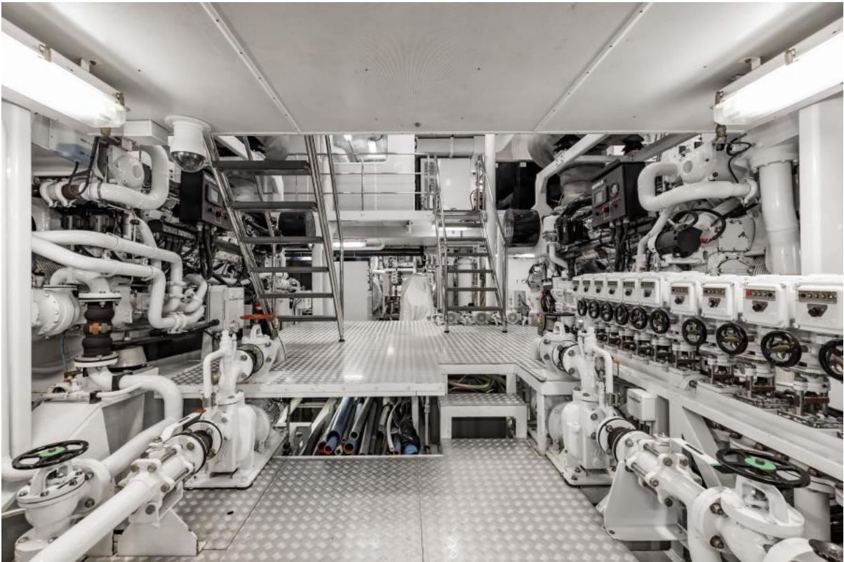
LAUREL 240'/73.15m Delta 2006/2014 Engine Room
