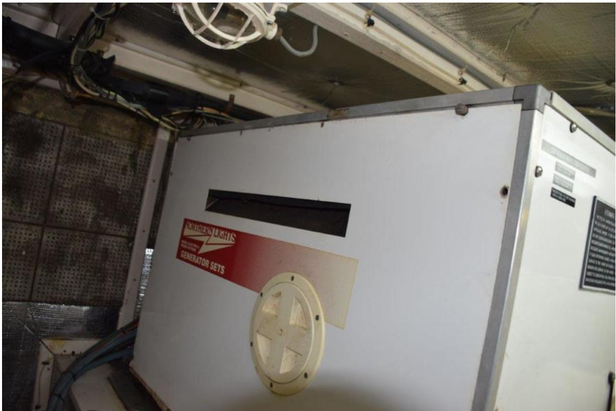
Northern Light Generator in Sound Shield
