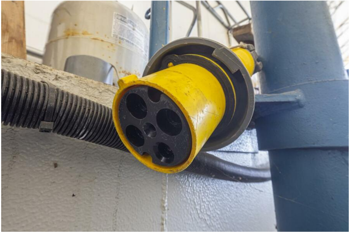
Shore-power 100amp Shore-power connection
